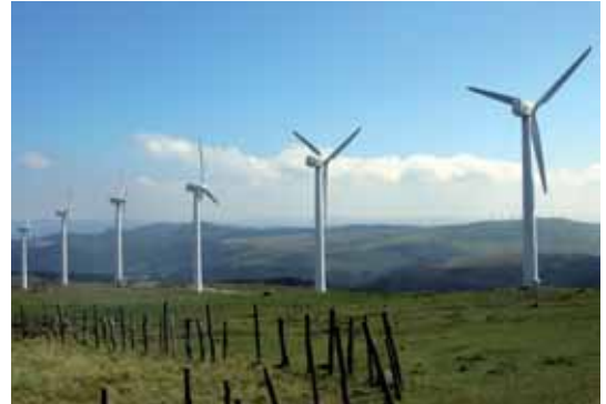
Renewable energies form an important part of local sustainability energy action plans
