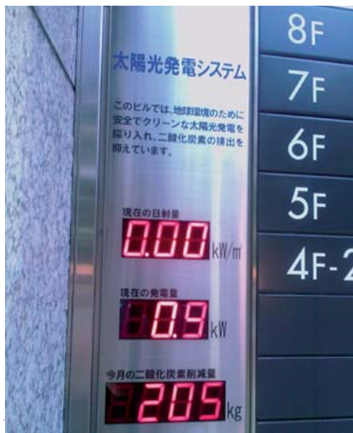
Solar information panel in a Japanese building
